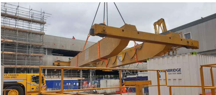
Crane unit removed safely and landed to ground level
