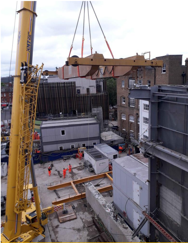
Crane being lowered
