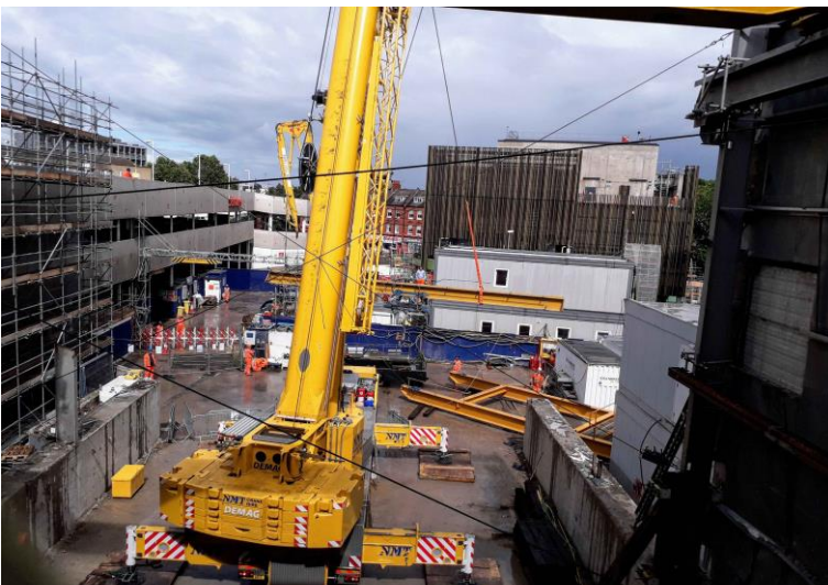
Mobile crane suspending and lowering the bridge beam
