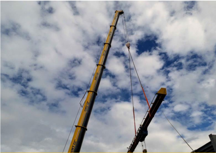
Lowering the bridge beam
