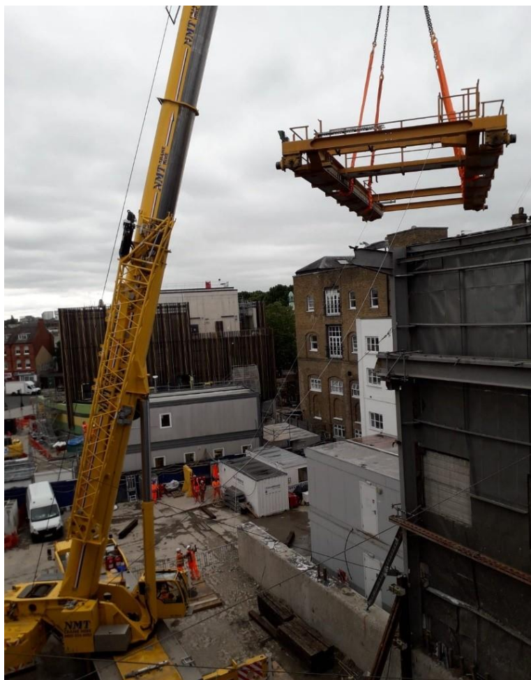
Mobile crane suspending and lowering the Kunz crane
