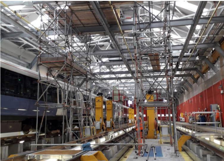
Twin tower scaffolding design
