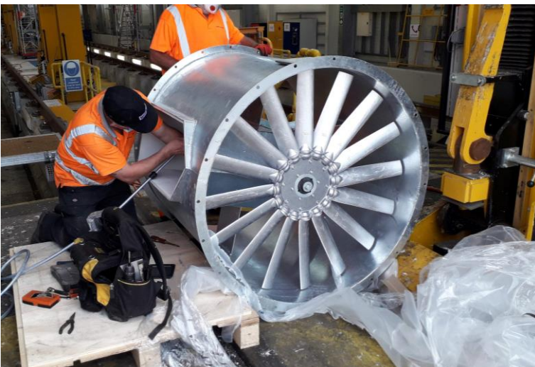
Preparing the replacement fan
