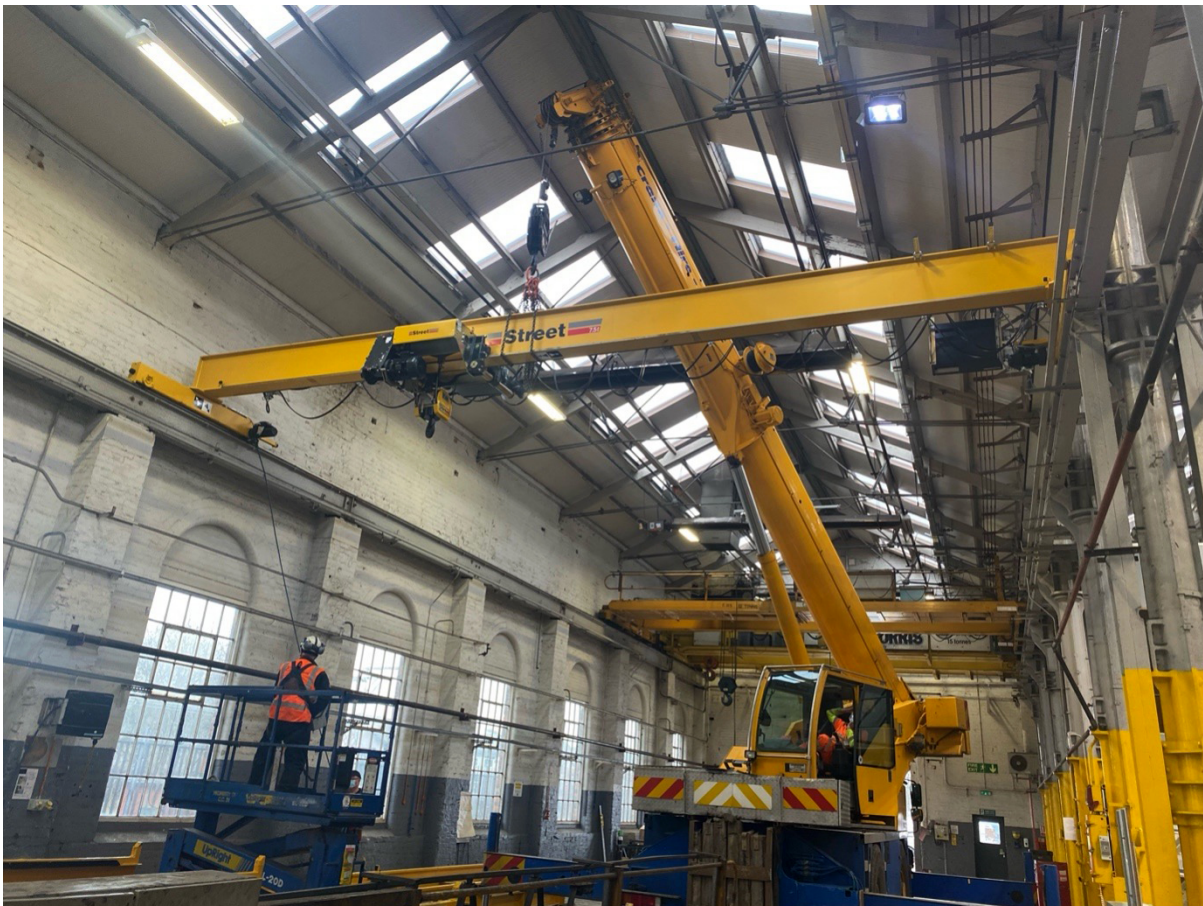
Installing the new overhead crane
