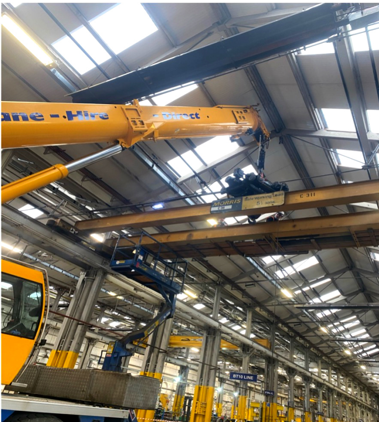
Removing the crab unit
