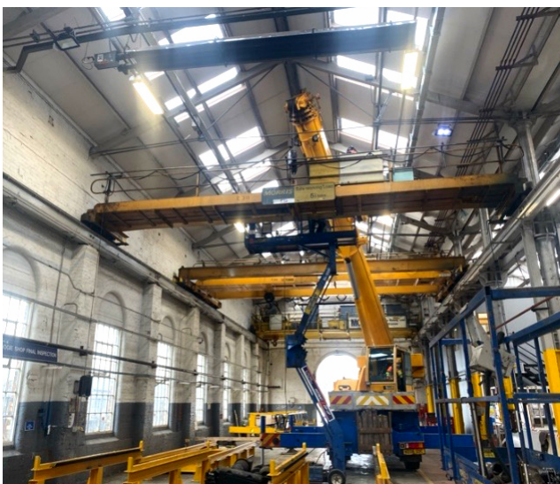
Lowering the main beam
