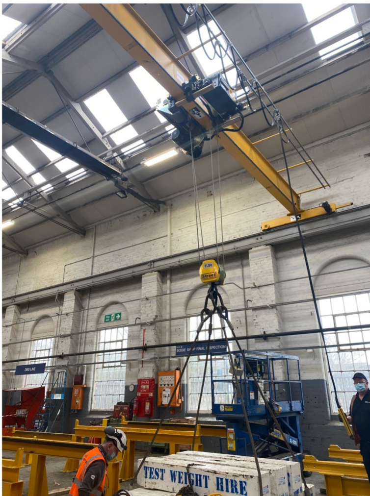
Proof load testing
