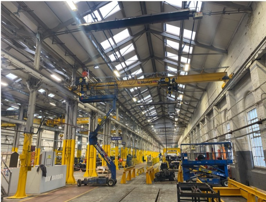
Adding collector arms to the overhead crane
