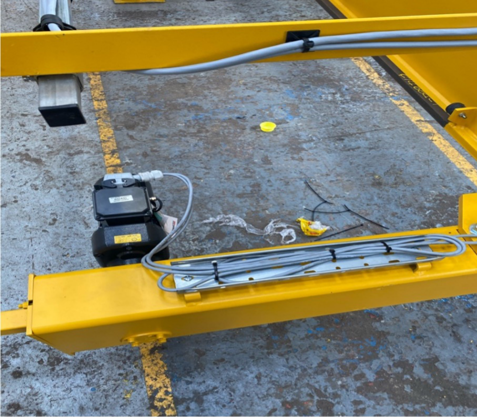
New crane being prepared at ground level
