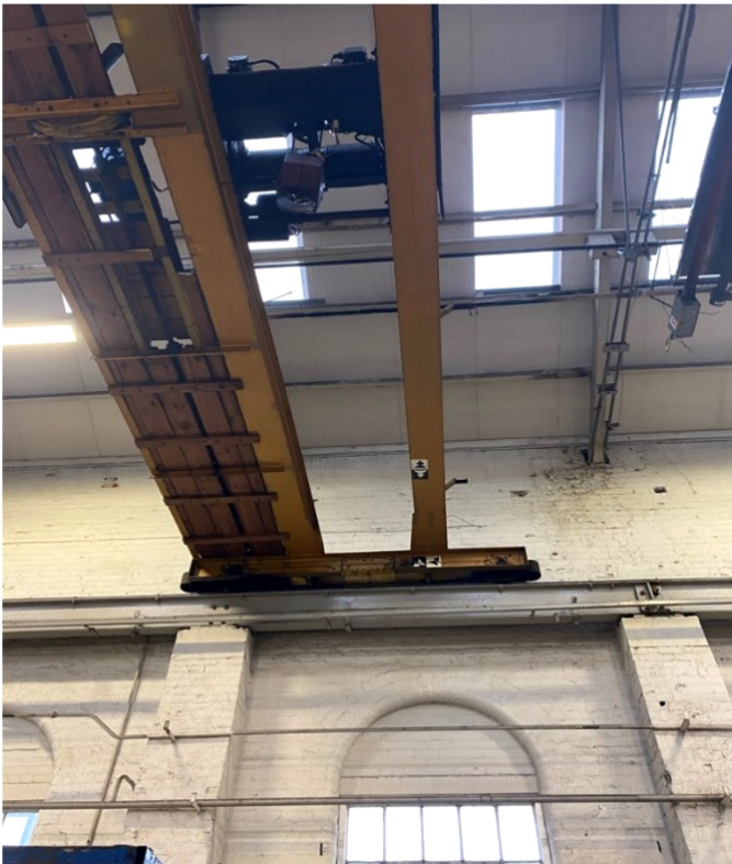
Splitting the beams
