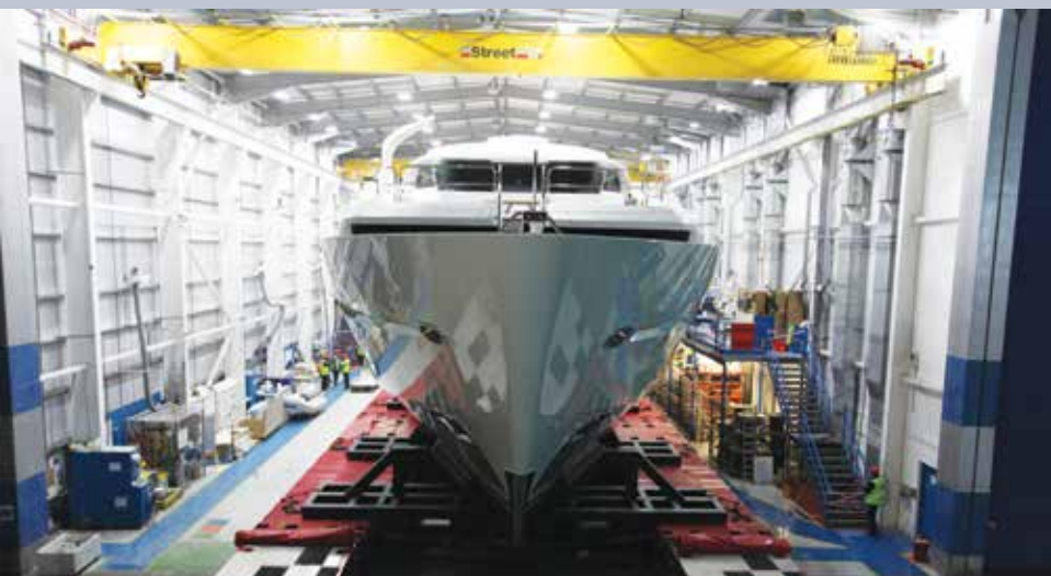
ZX overhead crane used during for the building of a £32M superyacht.
